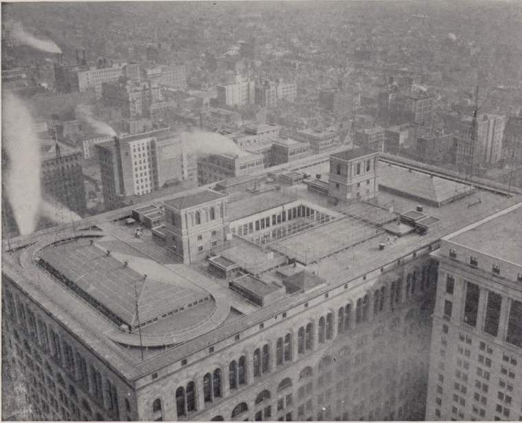
Fig. 30a.—Roof of the John Wanamaker store, Philadelphia, showing running track, basket ball and tennis courts.
